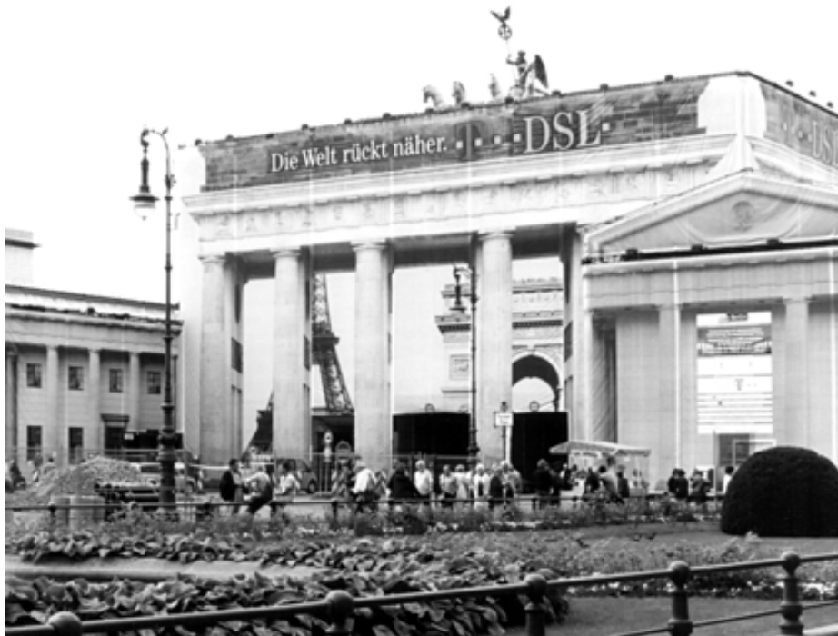
Figure 5: The image of the Eiffel Tower overlaying the Brandenburg Gate during restoration work. Berlin, 2003.
