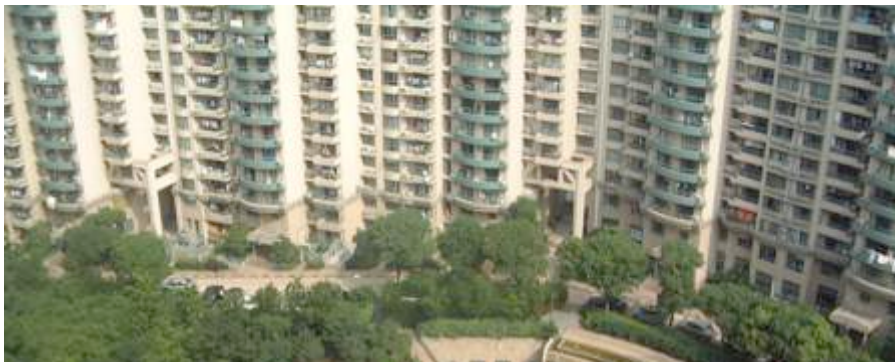
Modern residential blocks are on the constant rise in Shanghai and elsewhere in China.
