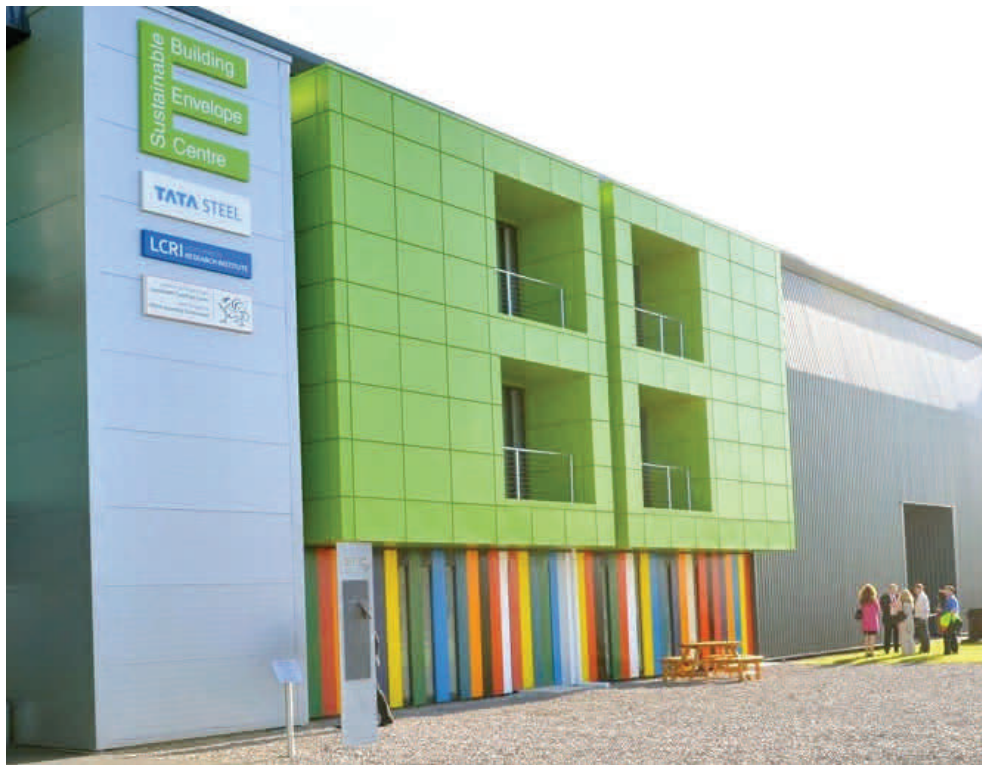
SBEC at Tata Steel's Shotton Works site in Flintshire
