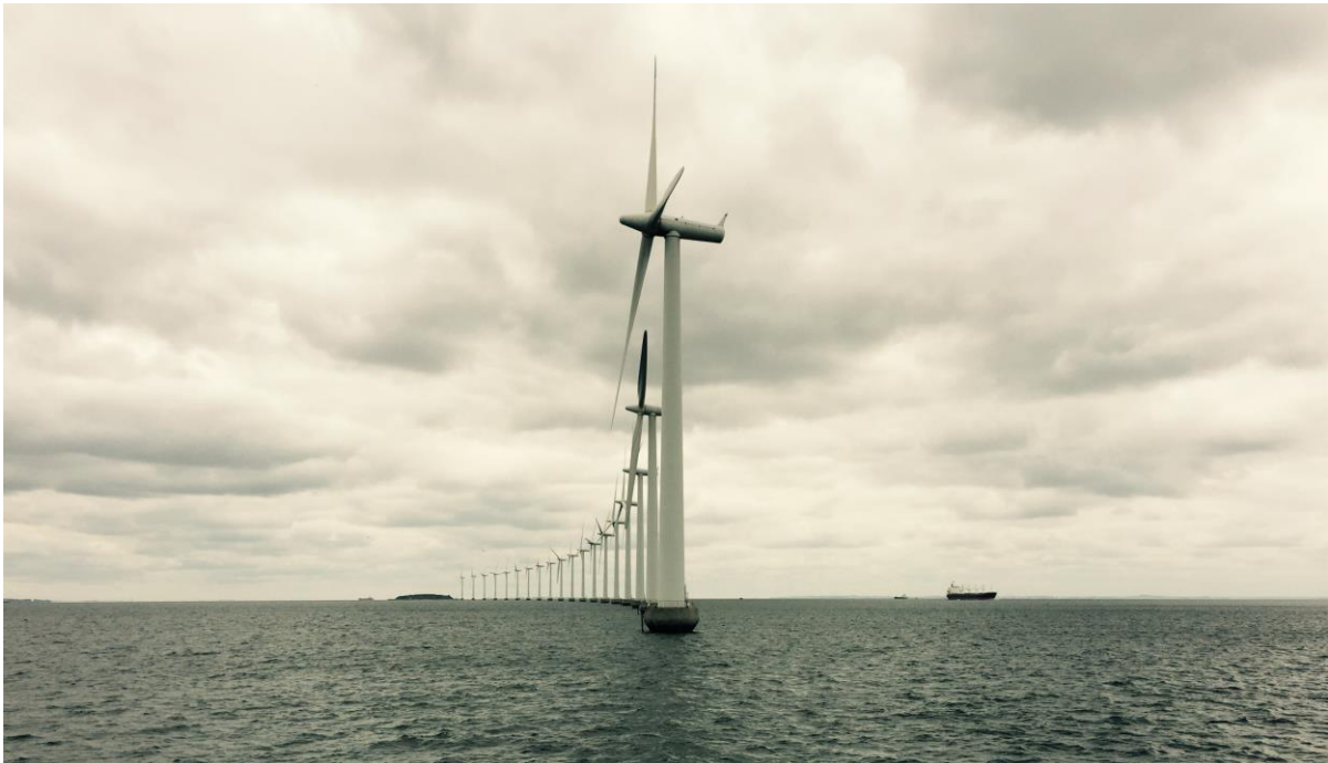
The Middelgrunden Offshore Wind Farm.
