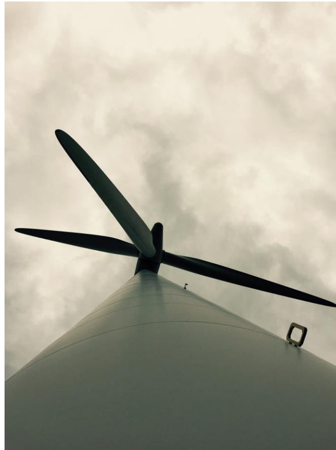
From the bottom of the wind turbine.
