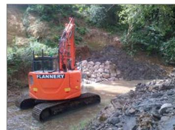
flows. The outfalls allow the dryside of the defences to drain without allowing high flows to outflank the embankment and flood properties. On the River Asker, at Lee Lane Bridge an embankment that had been undercut and slumped has been repaired.
